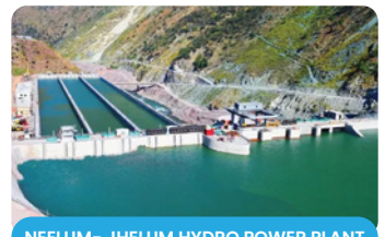
NEELUM- JHELUM HYDRO POWER PLANT
