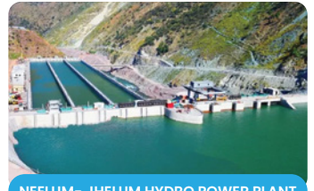
NEELUM- JHELUM HYDRO POWER PLANT
